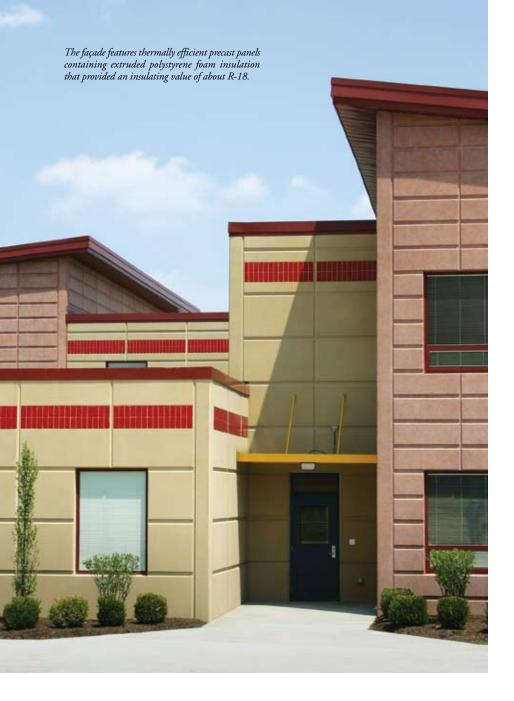
The school's initial brick-and-block design readily lent itself to conversion to precast concrete.
