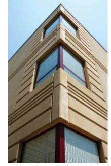
After embedded thin brick didn't meet budget requirements, designers used color, texture and articulation to create an aesthetically pleasing façade.
